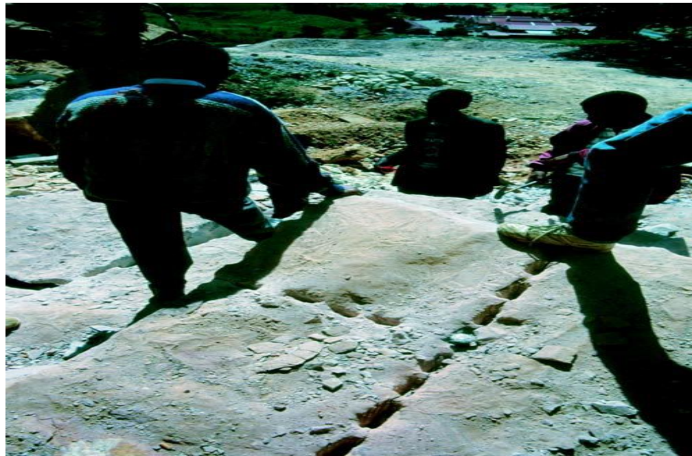
Figure 1. Wedging sandstone beds in the Ambo quarries.
