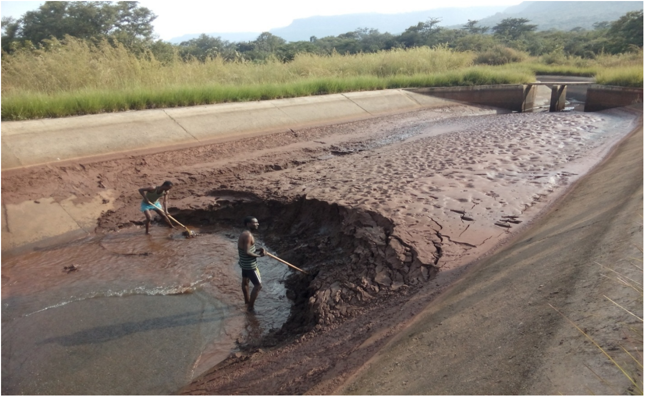
Figure 7. : Removal of Sediment Deposition from Settling Basin
