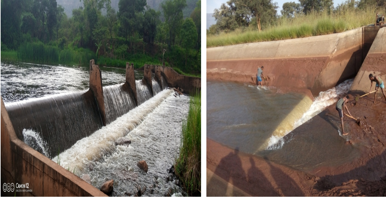
Figure 3. : Diversion Weir and Manual Removal of Sediments from Settling Basin
