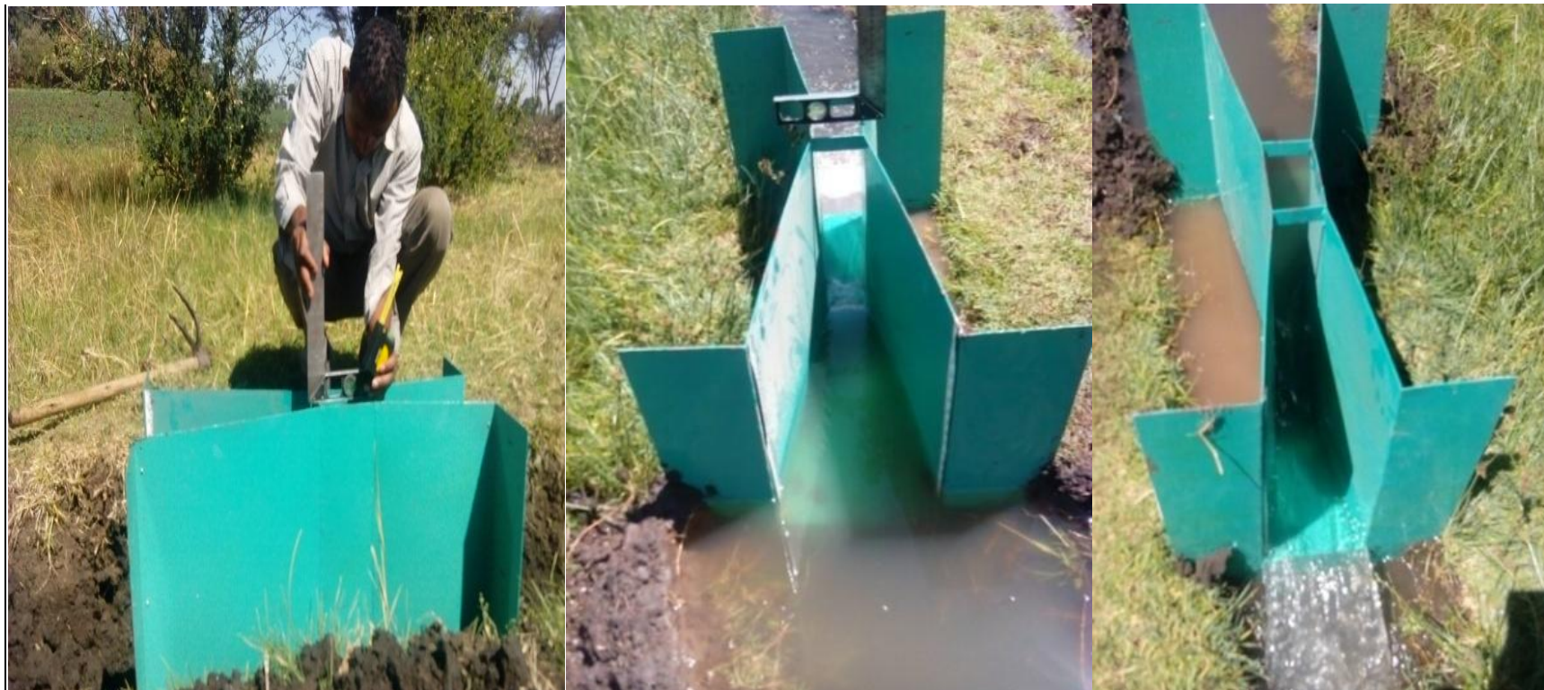
a. Parshall Flume Leveling
