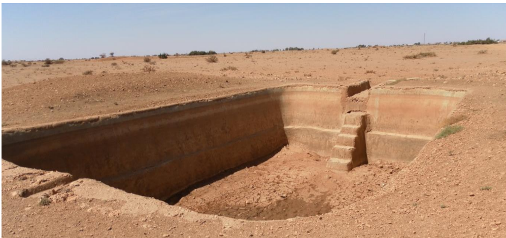
Figure 21: Unsuccessful Pond RWH Structure
